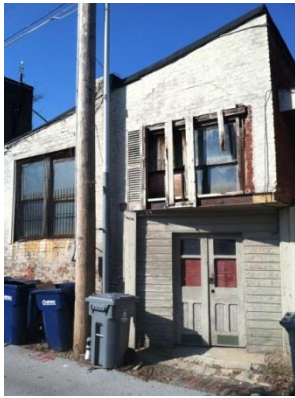
(Façade before Grant)
