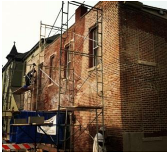
(Tuck Pointing in Progress)
